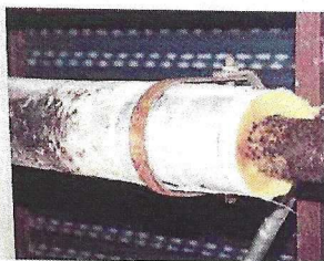
Glass fiber pipe insulation offers little resistance to the effects of moisture, including pipe corrosion and mold formation. Paper-backed all-service jacket (ASJ) is typically used as a vapor retarder over glass fiber pipe insulation. ASJ's delicate foil covering tears easily, allowing dirt, water and mold spores to enter the fibrous insulation. The paper backing on ASJ also provides a nutrient source for mold.
