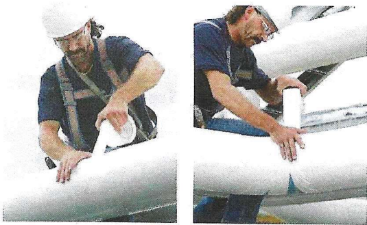
Saran Vapor Retarder Film and Tape provide continuous protection from water vapor drive, even at elbows and fittings.
